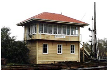
1: Bendigo Box A where it originally stood at the Bendigo Railway Station. Unknown Photographer, 15/8/1989, www.stationspast.net/.../bendigo-area/bendigo-a-box/
