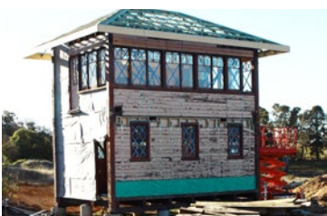
4: The signal box as at July 4, 2024
